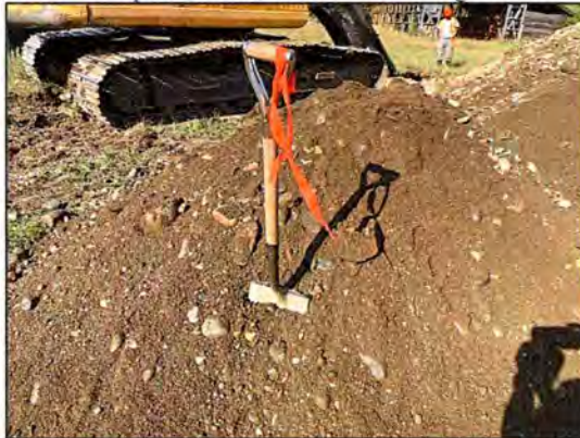
Test Pit 23-08 Spoil (Clean, gravelly sand 4.6-6.0m)
