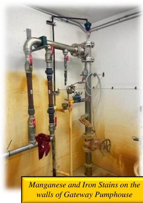
*Manganese and Iron Stains on the walls of Gateway Pumphouse*
