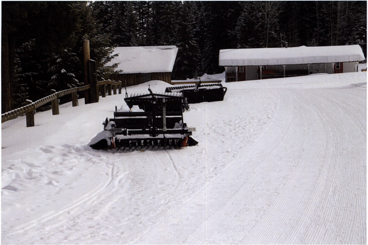
These are the original buildings with the building on the left being the original building brought from the 108 North Entrance where we had a series of trails which we ran races on. The building on the right was donated by Weldwood for our First Aid and storage.
