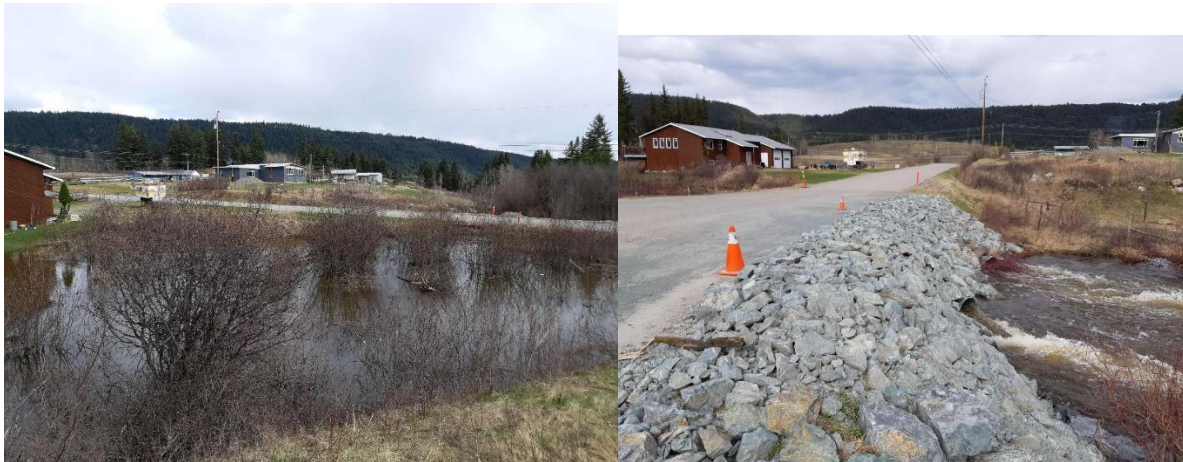
Figure 6 – Water flow exceeding culvert capacity, backing up water and causing flooding. (Photo Credit – CRD)
