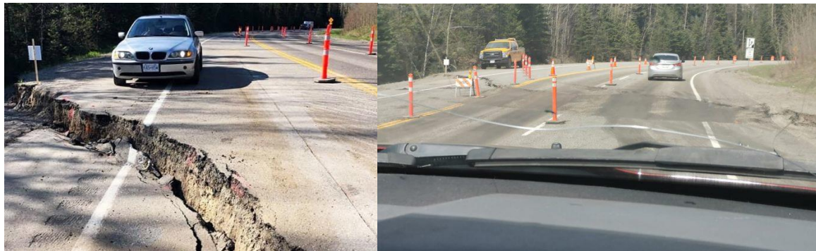
Figure 3 – Head and toe of rotational landslide often creates bump on roads – Hwy 97 @ Cottonwood River. A similar bump commonly appears at toe of Hodgson Rd slide on Hwy 20 in Williams Lake. (Source – Quesnel Observer & MyCaribooNow.com)
