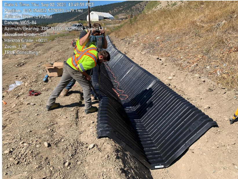
Installing “Smart Ditch” Earth Anchors.
