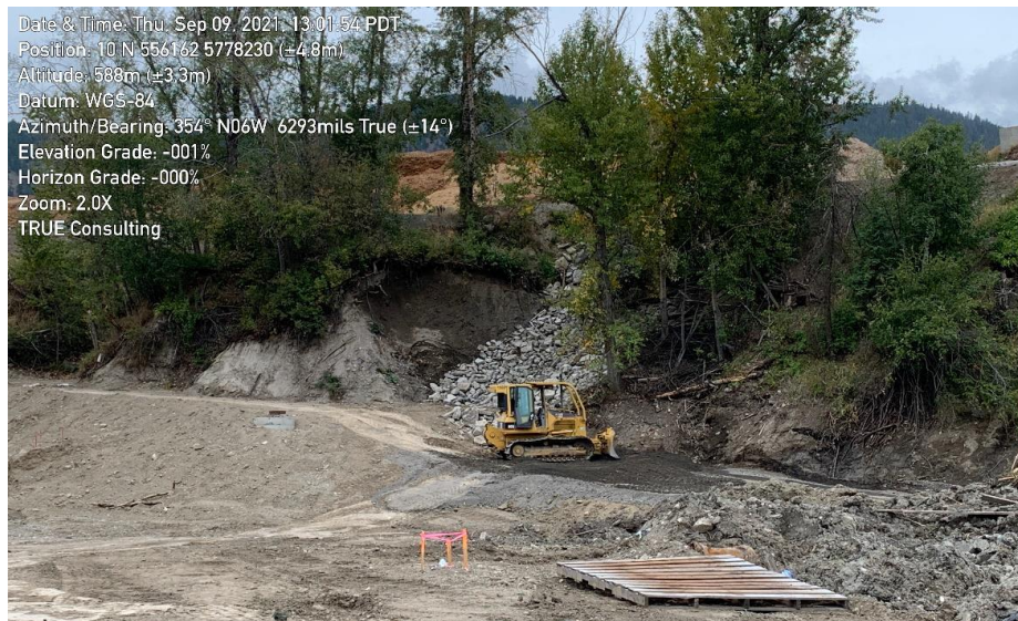
Using Concrete Waste for Berm Construction.
