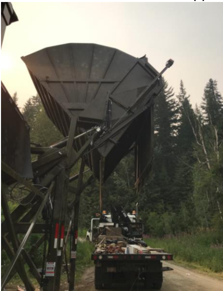
One of the new bins at Horsefly transfer station being tipped.
