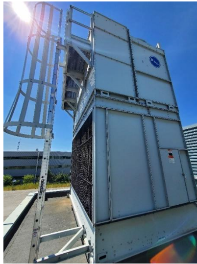
Figure 5: BAC Evaporative Condenser at CMRC
