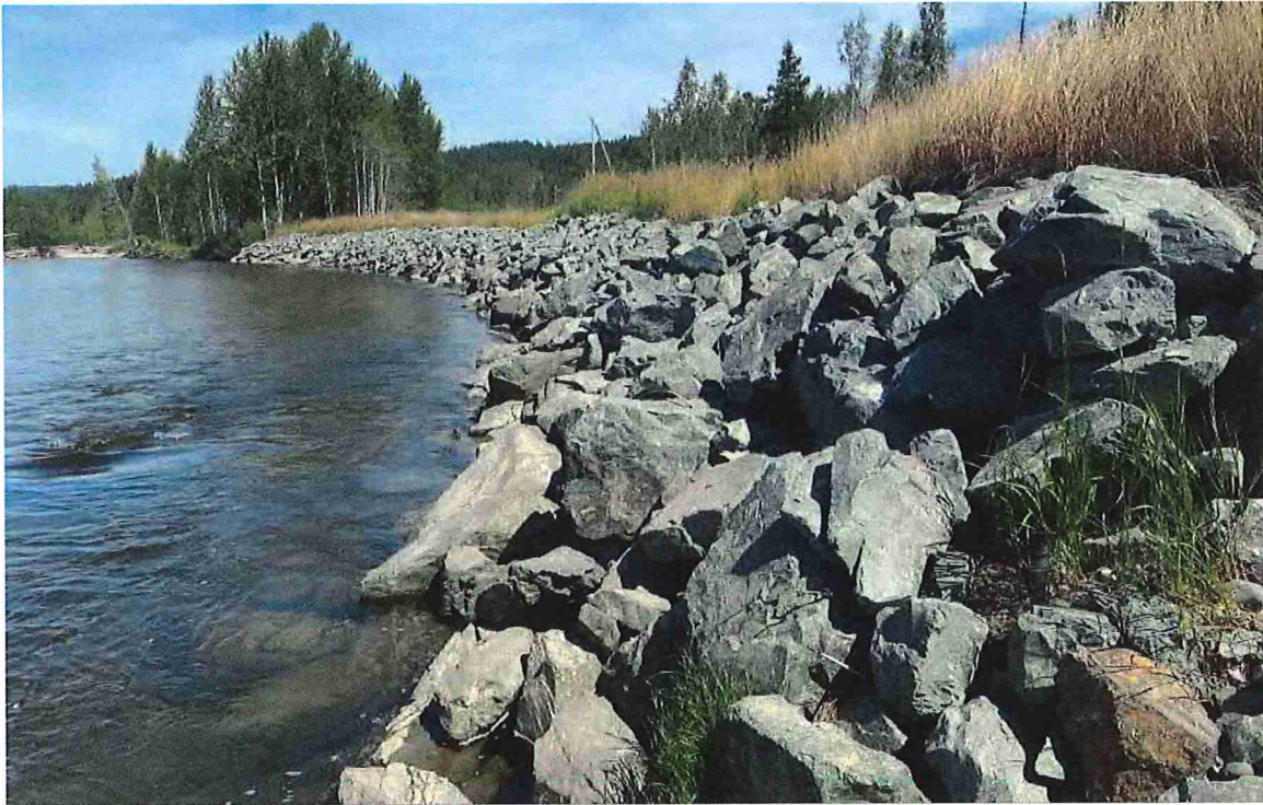
Quesnel-Hixon Road Protection - Riprap (Looking North)
