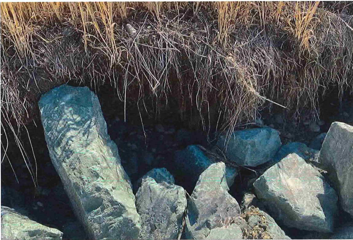
Quesnel-Hixon Road Protection – Riprap Top Scour
