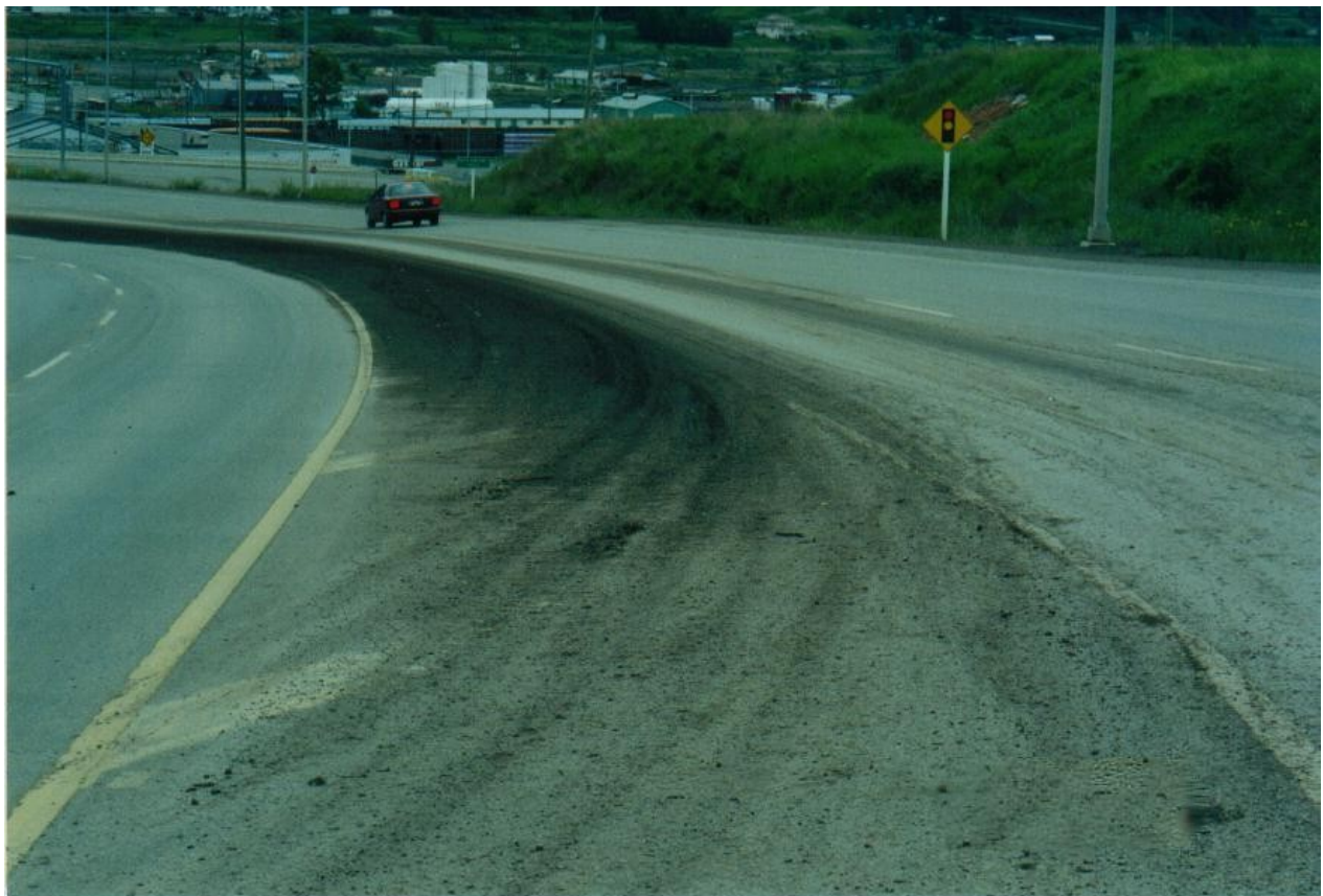
Soil material being tracked from an unpaved roadway to a paved surface contributes to elevated PM 10 values in Williams Lake.
