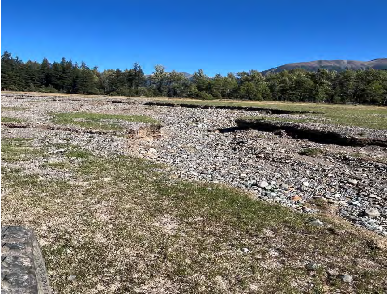
Fig # 16 2024 Unmanaged same location ( different view upstream) 1 year later
