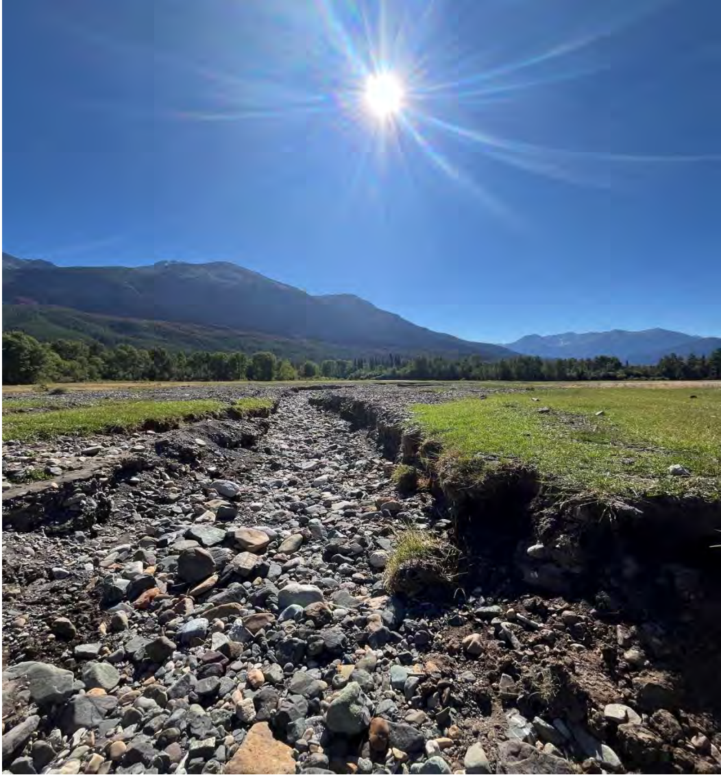
Figure # 17 Aug 2024 Full View of Burnt Creek damage
