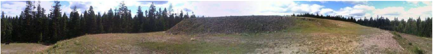
Photo 4. The upper lift of Landfill located in the northern portion.
