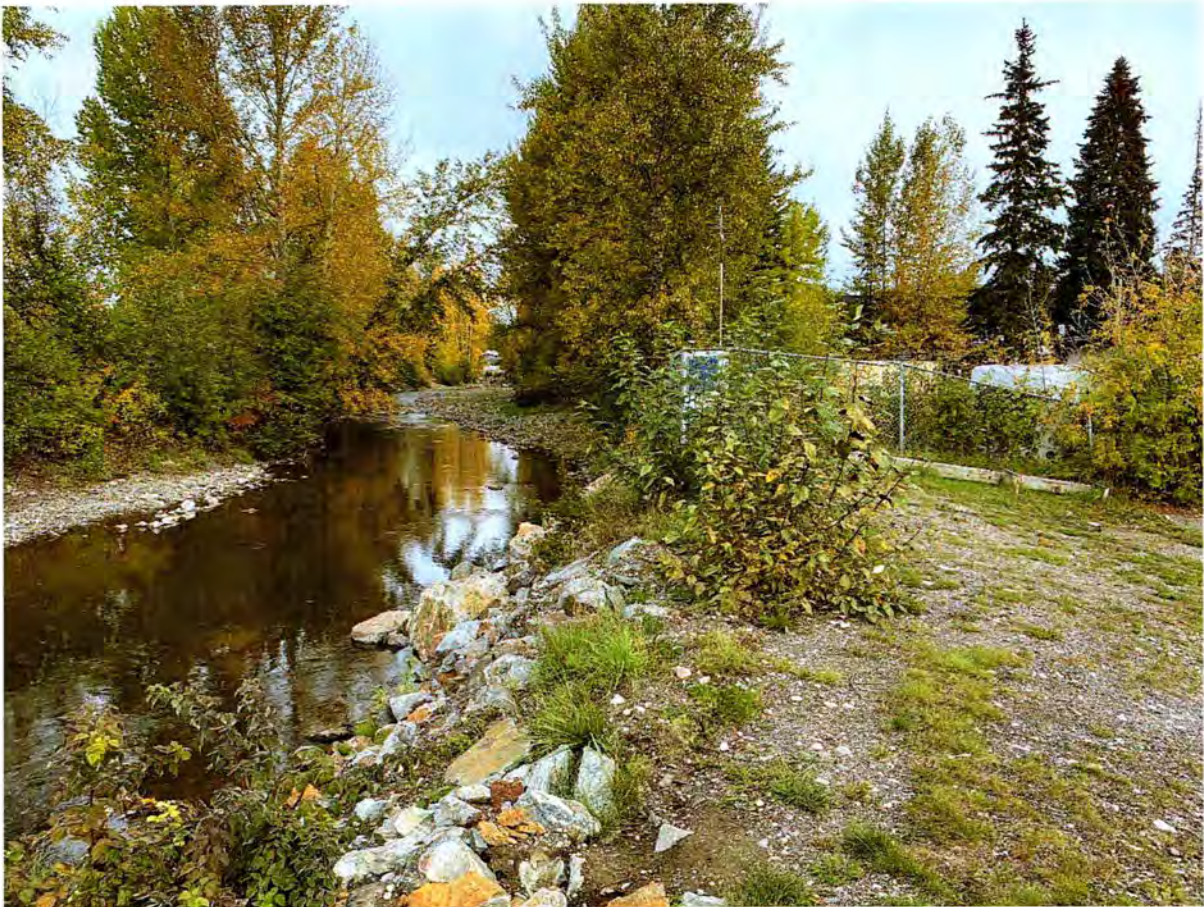
Photo 12. Baker Creek upstream of the Marsh Drive Bridge, looking upstream. Photo taken on September 28, 2024.
