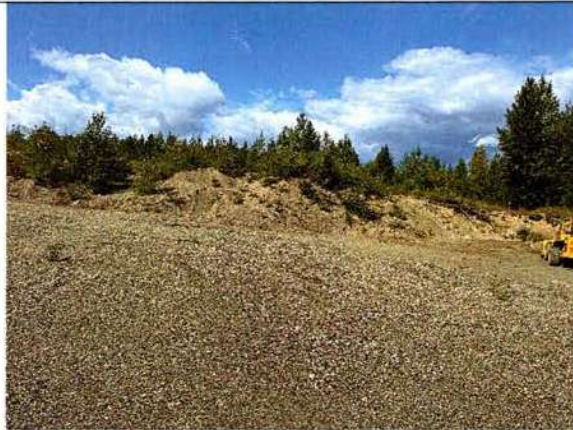
Photo 1: Existing pit showing disturbance looking north.
